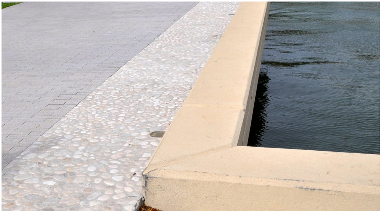
Figure A.5: Example of Traditional 7ft Sea Wall Bulkhead / Sea Wall Cap
