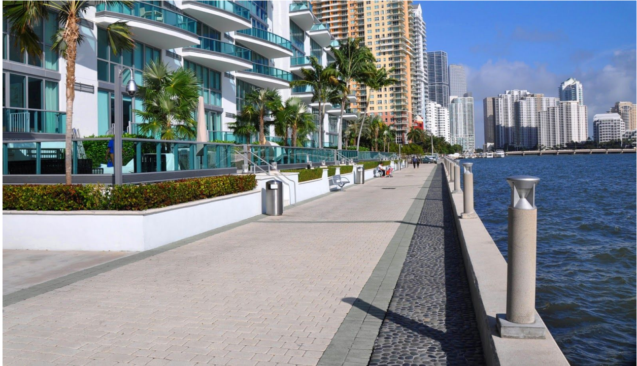
Figure 3: Example of Traditional 7ft Sea Wall with Baywalk
