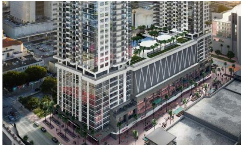
Developed by CIM Group in partnership with Falcone Group, the tower marks the latest addition to the $2 billion mixed-use project.
