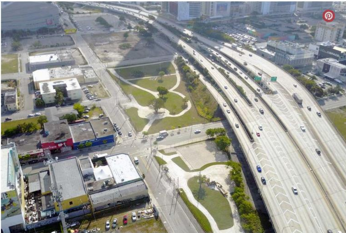
Rendering of the Omni Park in downtown Miami | Courtesy of Omni Park
