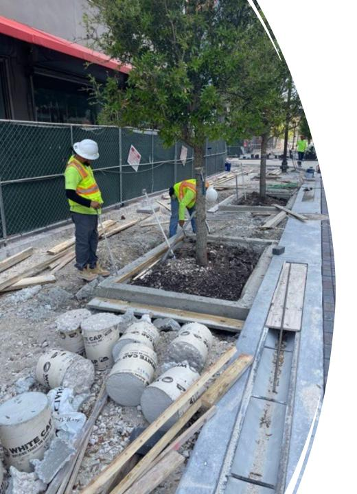
Removing forms from tree grate curb supports
