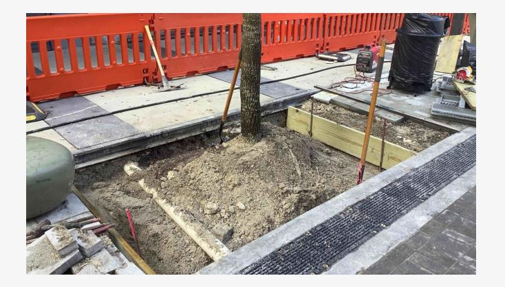
• Grading material and installing forms for tree grate footer.
