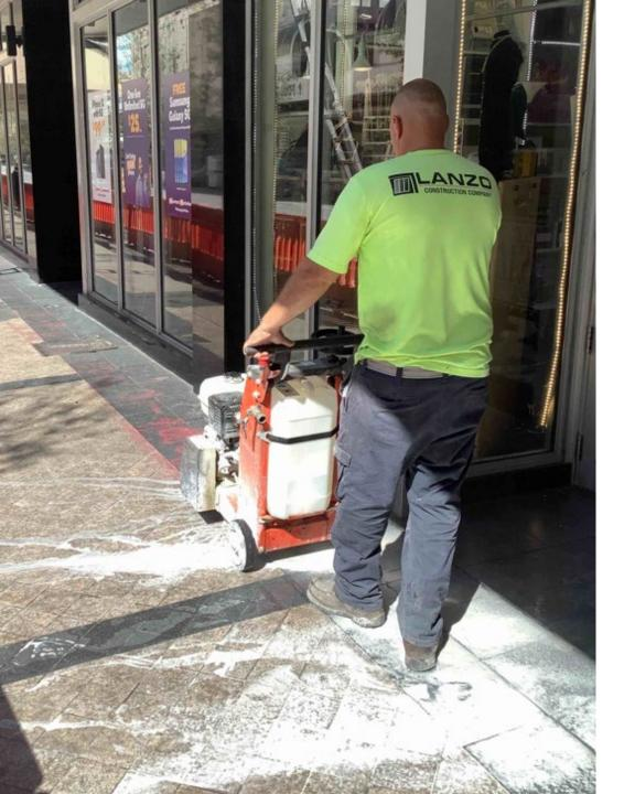
• Saw cutting sidewalk in preparation of sidewalk demolition.
