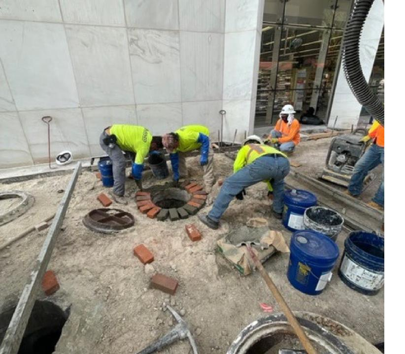
Utility Manhole & Valve Adjustments in Preparation for Sidewalk
