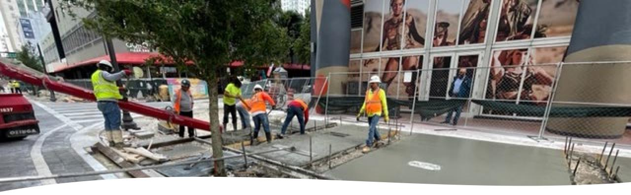
• Casting of New Exposed Aggregate Sidewalk
