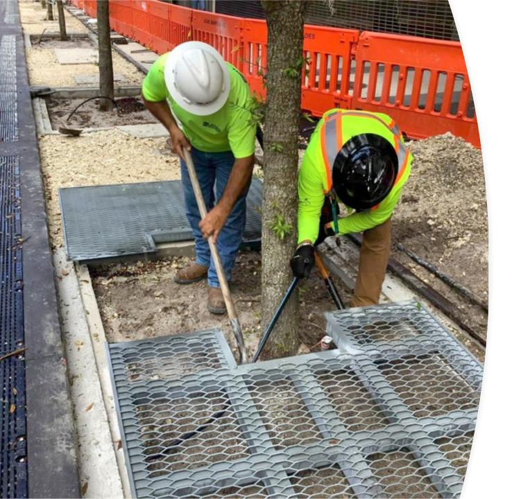
• Installed grates, filter fabric, and sand for tree pit area.
