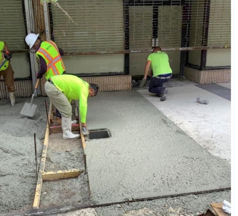
• Placed concrete for sidewalk on north side of section D.
