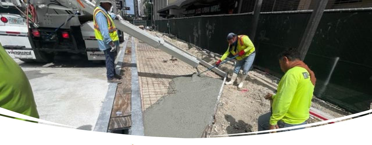
• Casting of 8" concrete slab valet area
