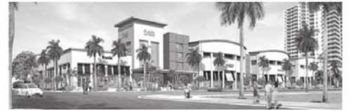
New Publix is to have 8,000 SF of other retail space facing Biscayne Blvd, including a bank.
